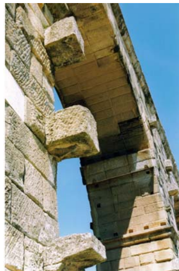
Stone blocks without mortar, Pont du Gard, Nimes
