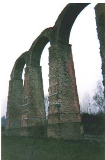
Stone masonry, Aquil Terme, Italy
