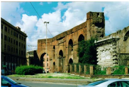
Brick faced concrete, Nero's branch, Rome
